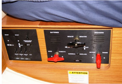
Jeanneau 39DS - Battery Switches
