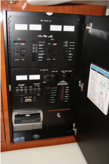
Sea Ray 395 - Electrics Panel
